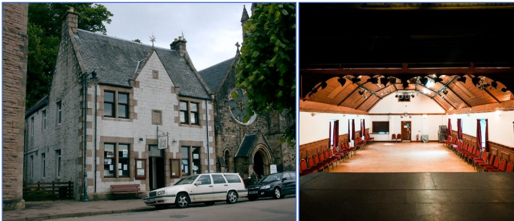
Figure 2.1: External and Internal Appearance
