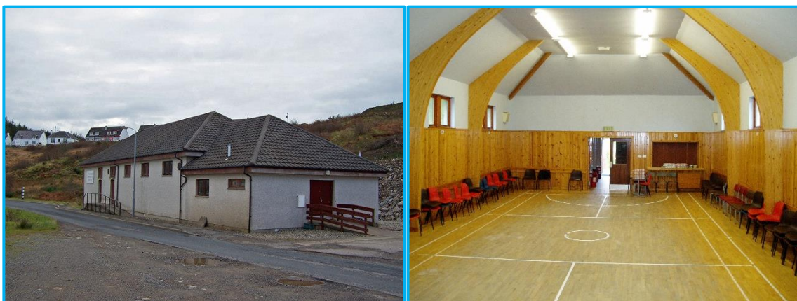
Figure 3.1: External and Internal Appearance
