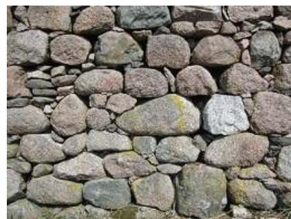
The dry stone plinth should follow the local vernacular style, recognising that this style does change across Mull (Ross area pictured right). The plinth should be low and angled. It is envisaged that this plinth is only around 400mm in height at the front and around 600mm at the rear. The panel will need to be securely fixed to a solid central column within the drystone structure.
